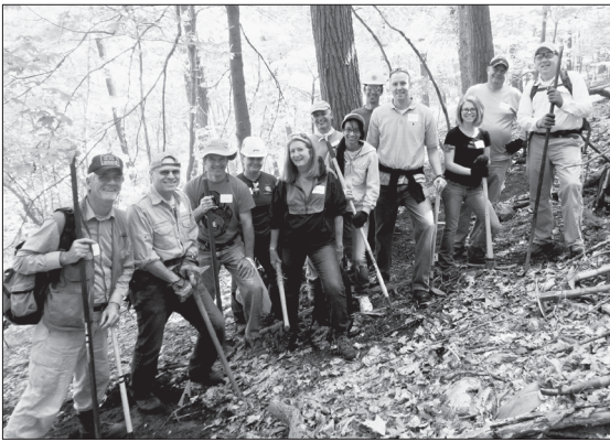
Volunteers building the new trail from the Museum to the trails in Black Rock Forest
